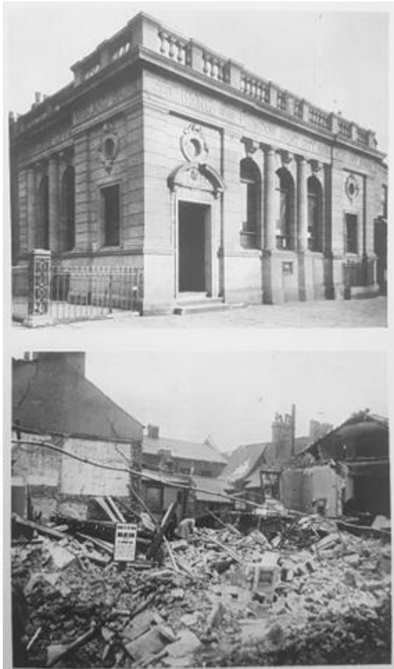
The Midland Bank at Witham, Hull, before and after a raid.
