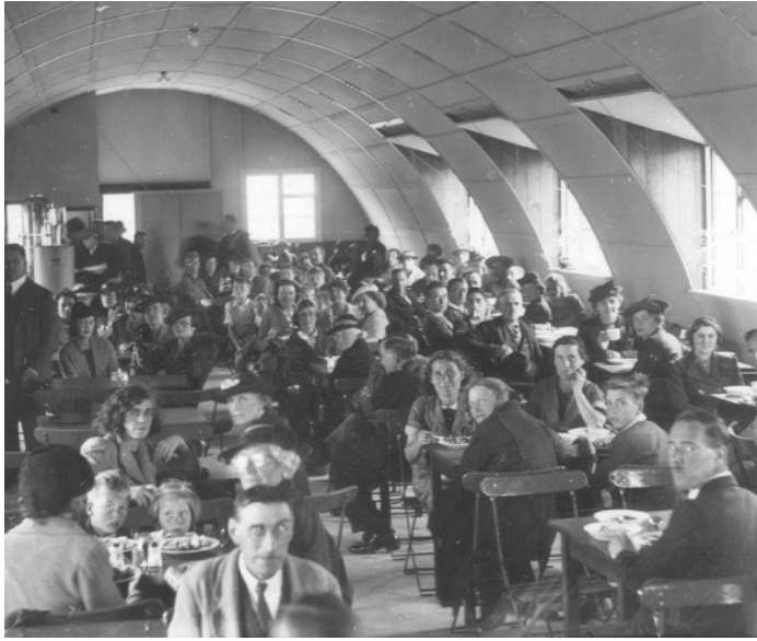
British Restaurant in Portsmouth
