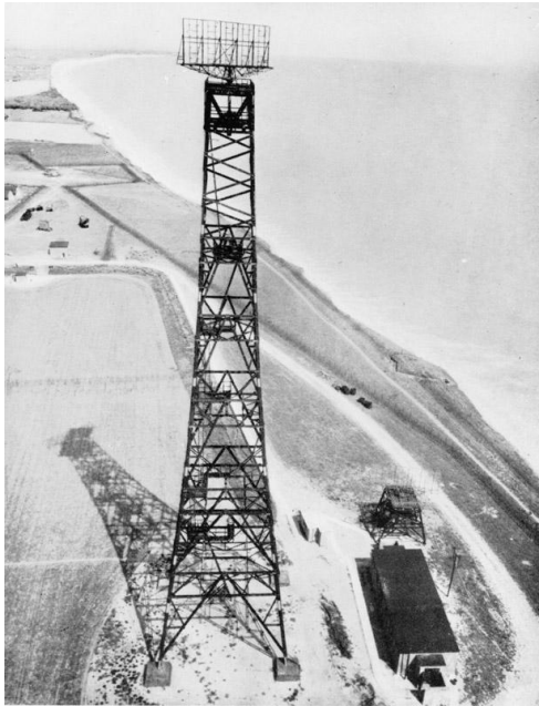
Left, A view of a 'Chain Home' Low Station, used to detect and report low-flying aircraft. [This type of radar mast helped to secure Britain's victory in the Battle of Britain]. Below, WAAF radar operator Denise Miley, plotting aircraft on a receiver at Bawdsey Chain Home station.
