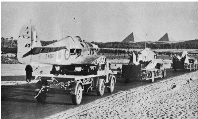
Several RAF aircraft seen in one convoy heading to Cairo where they would be assembled and despatched to the combat area. We can see that these were involved in accidents and damaged during the long journey. The Hurricane nearest the camera has suffered damage to its tail section and panels are missing from the fuselage side and engine area.
