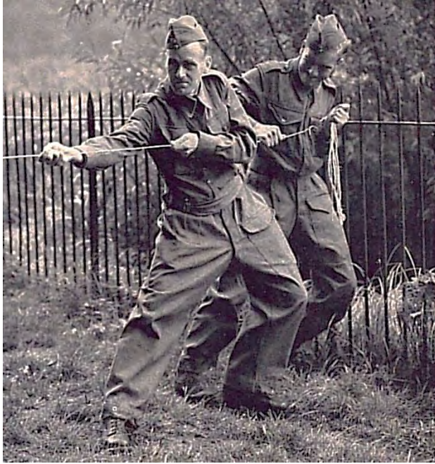
Stringing a wire across a road.
