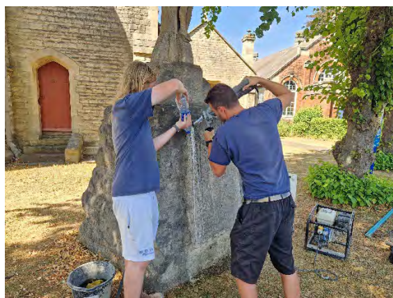
Drilling the old plaque commences
